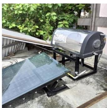
Gambar 3. Alat Solar Water Heater
